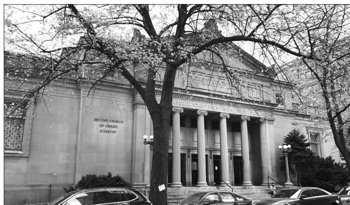
The 2nd Church of Christ Christian Science building at 2700-2717 N. Pine Grove Ave.
